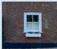
Sash window and white decoration around the window
