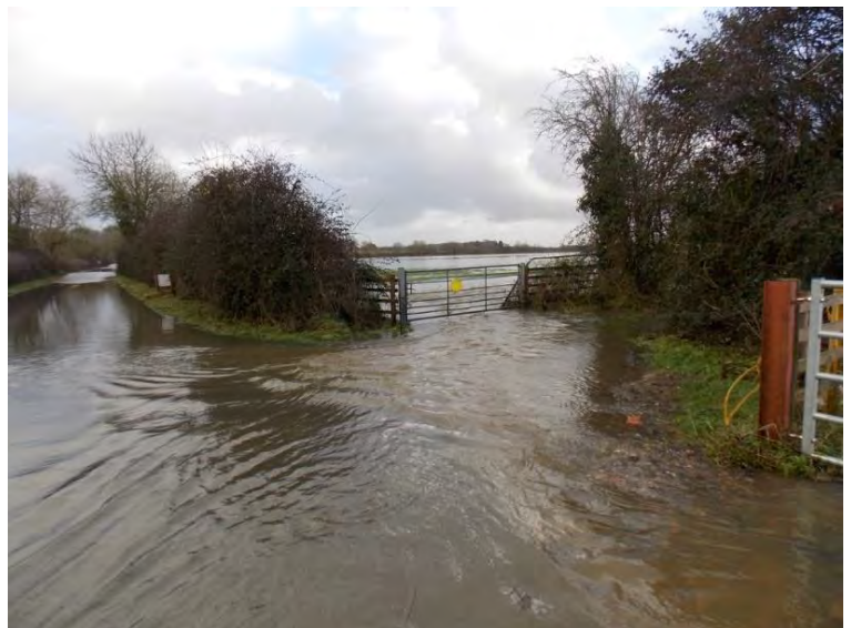
Figure 1. Flooding in Mill Lane from river overtopping
