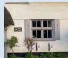
Window with external shutters
