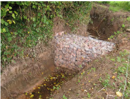
Gabion basket, immediately after construction.
