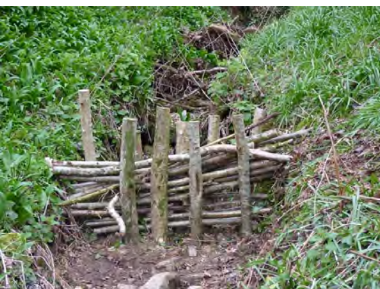
Leaky barrier using hazel bundles
